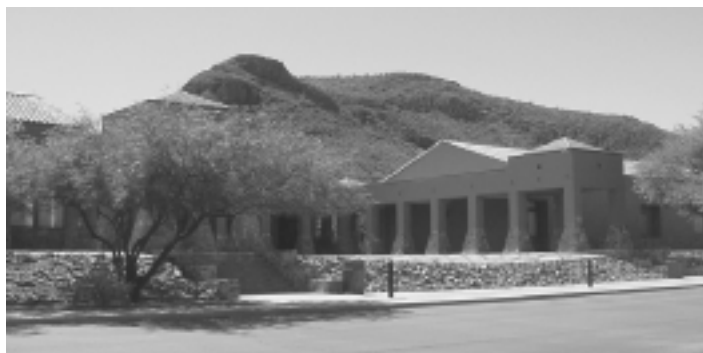
Caterpillar facilities in Tinaja Hills near Tucson
