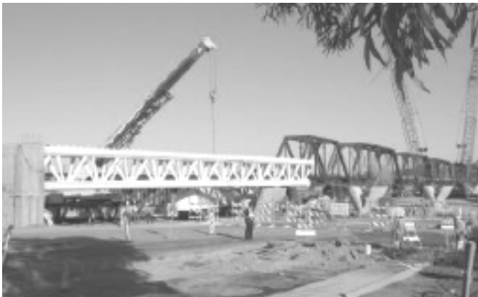
Tempe Town Lake Bridge under development for the Valley Metro Rail.
